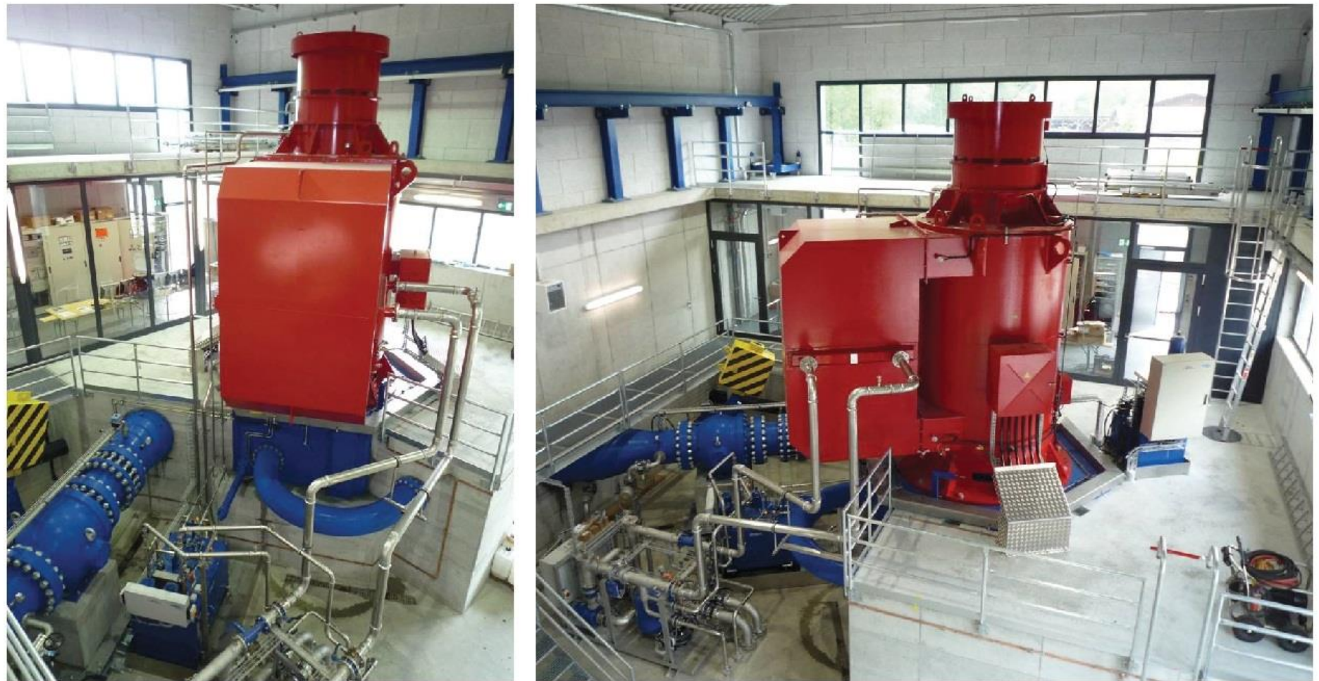
Figure 13: Photo of Similar Sized Pelton Wheel Generator Installation
