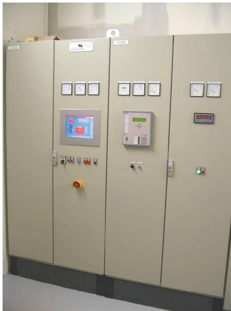
Figure 7-21: Example of Control Panel and Mimic Diagram Display
