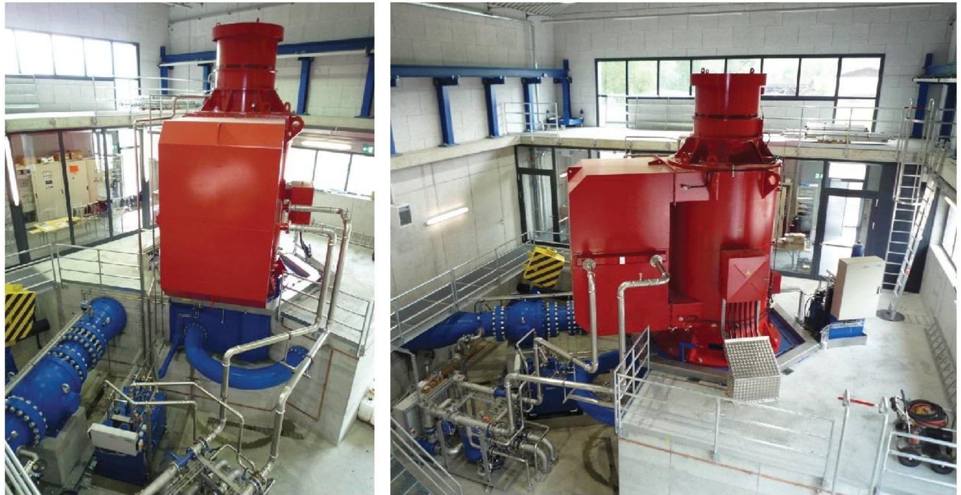
Figure 7-19: Photo of Similar Sized Pelton Wheel Generator Installation
